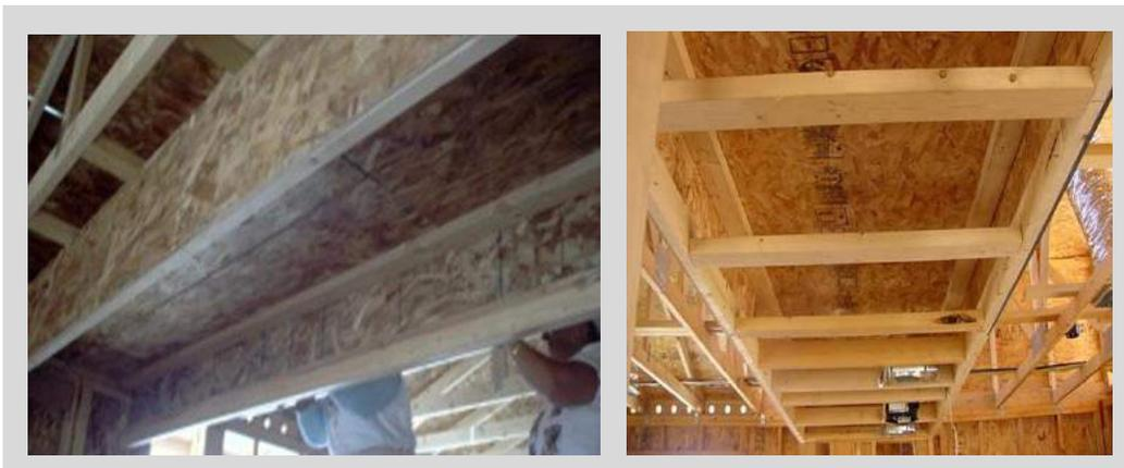
Add 2x4 blocking between the bottom 2x4's every 24" O.C. (adjust spacing as needed to avoid lights or fan) to ensure proper width. **Do not install OSB on the bottom of the soffit.**
