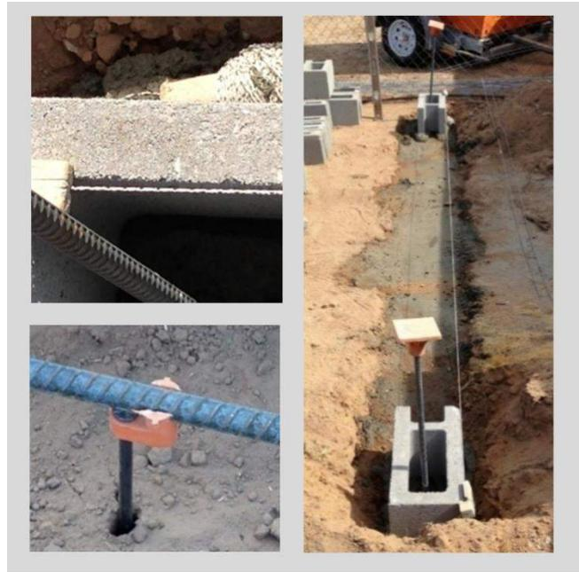
Once the leads are completed, we start building the wall in panels (the sections between pilasters), usually one panel per bricklayer.
