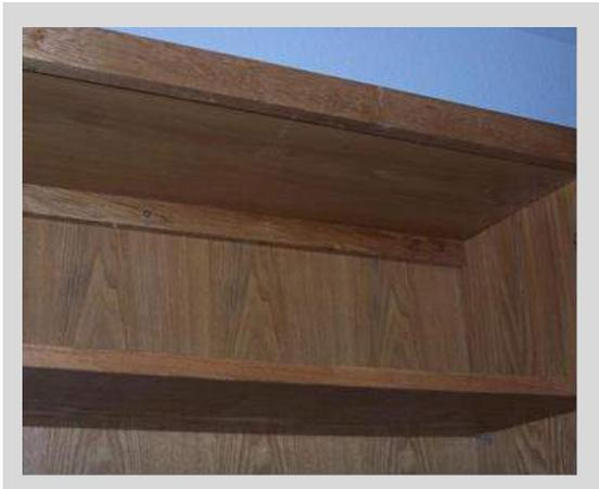
8. At this point install any needed filler strips between cabinets and end walls.
