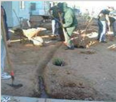
9. All copper will be installed at the correct grade and tested by staff prior to landscaping, as will the entire manifold/valve assembly (this includes the filter, pressure reducer and adapter for the drip tubing). Do not make any changes to any part of the assembly installed by staff. All you will need to do is attach the drip line to the completed assembly and install the valve box so that it sits 3" above the dirt to allow for the granite.
