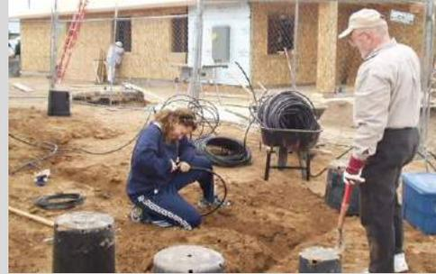
**11.** Run the main line through the sleeve under the driveway and through the block wall and stub it out in the back yard. Also run the main line through the block wall and stub it out on the valve box side of the house.
