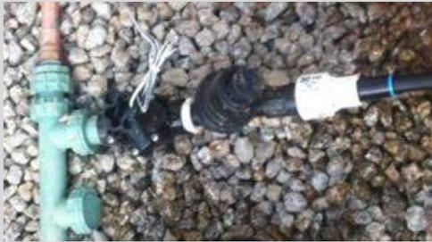
**12.** All plants get one 1-gallon emitter each. The emitters are installed directly into the main line, and the mini tubing is run from them to the plant. MINI TUBES CANNOT EXCEED 3' IN LENGTH.
