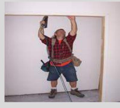
Install the track in middle of the header. Use ALL screws provided for the track.
