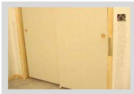
To ensure the doors are hung properly, you MUST locate the solid block provided at the edge on one side of door to mount inset door pull. These blocks must be on the outside edge of the doors when they are hung.
