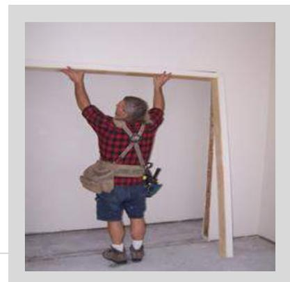
7. Once you have determined the jamb lengths, verify that they will fit in the opening, and then cut to length.
