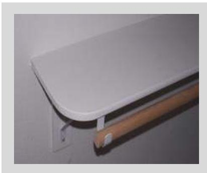
Round off the floating corners of the lower shelf using a coffee can to create the radius. Cut it with a jig saw and clean up with a belt sander. Just remember to extend the shelf enough for the shelf bracket to clear the round off.
