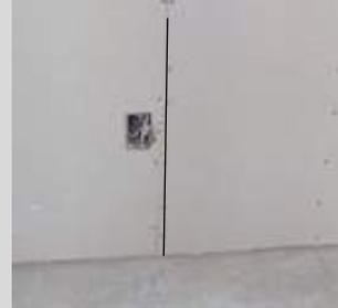
*Avoid joint breaks next to outlets, switches.*
