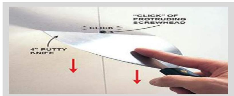
Please be very thorough doing this recess check as the protruding heads damage the finisher's tools.
