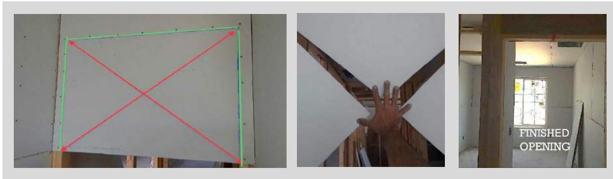
1. From the back side make a nail hole in each corner. Then score along the three edges of the frame with a utility knife and score an "X" across the entire opening.
