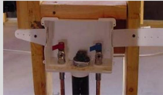
Block around the dryer vent box. Install a piece of blocking across the top and a piece down the side.
