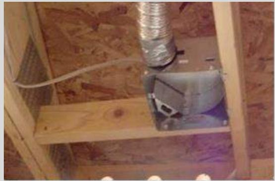
Block behind icemaker water box. If the plumbing line runs vertically, notch the top block as needed to fit around the line.
