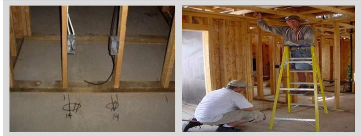
Marking Fixtures: Use a marker to indicate every electrical outlet, plumbing outlet, vent, ceiling fan, smoke detector and ceiling light. Measure down from the middle of the wall fixture to the floor and write down that number on the concrete. **Remember to use pencil on exposed concrete.**
