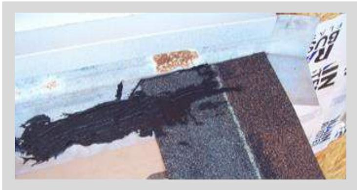
We are no longer using metal valley flashing on our roofs. The new procedure is done with shingles only and is detailed in the section on shingling. At this point all that needs to be done is to run a piece of underlayment down the valley.
