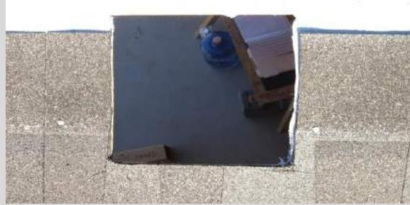
4. Turn the vent right side up and using your marks as a guide set it in place. When you are satisfied with its location, press down the areas over the tar beads.
