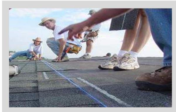
Please note that in the preceding photo, the volunteers are working from above the shingles, not standing on them. This is imperative in hot weather and when the direct sun has softened the shingles. **Excessive traffic (particularly the twisting of feet) will damage the shingles.**
