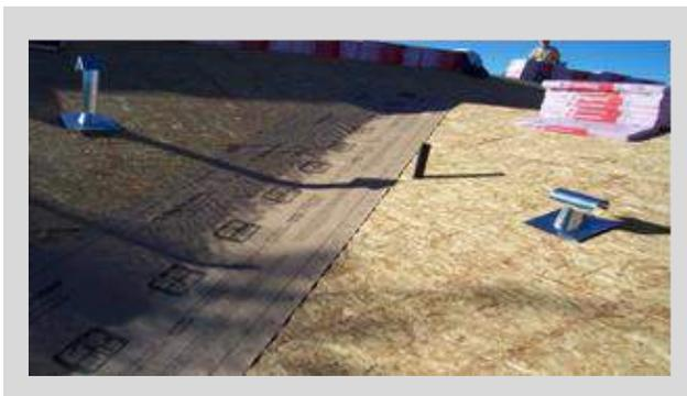
All roof penetrations require a galvanized metal roof jack. At this point verify once again that the proper jacks are on hand. These will be installed over the underlayment, and in between the layers of shingles. Install a second piece of underlayment (about 2 feet wide) over the top half of the jack flashing and extend it up under the next highest joint for further leak protection. Do not install the jacks until shingle installation.
