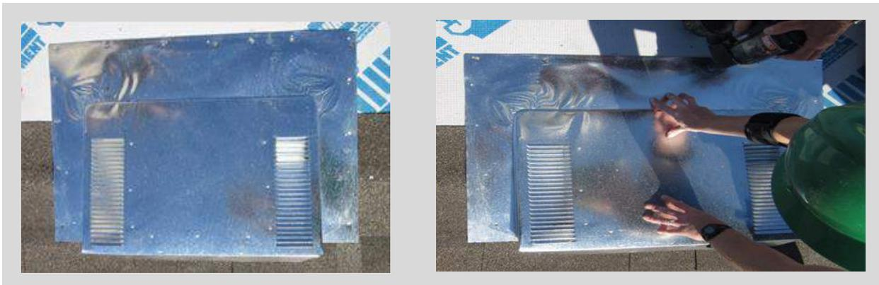
5. Using long roofing nails at 4" o. c. nail the top and both side edges through the area of the outer tar bead.
