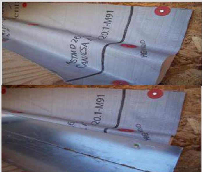
Attach the L flashing to the flashing nailer with 1- 1/4" roofing nails along the top edge of the metal. Always try to keep the nails as far from the bend in the L flashing as possible (Nail high). Do not nail into roof.
