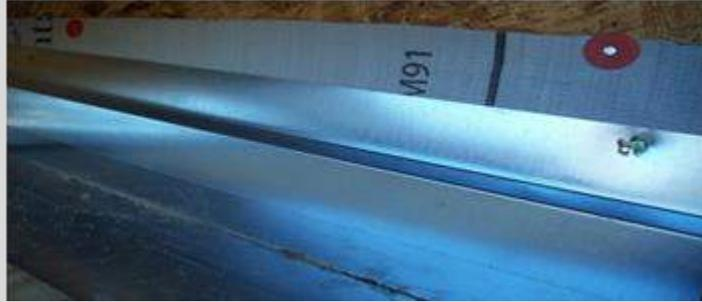
7. Install the upper leg of the Z flashing to the vertical wall using 1- 1/4" roofing nails so that the flat of the Z sits on top of the flashing nailer.
