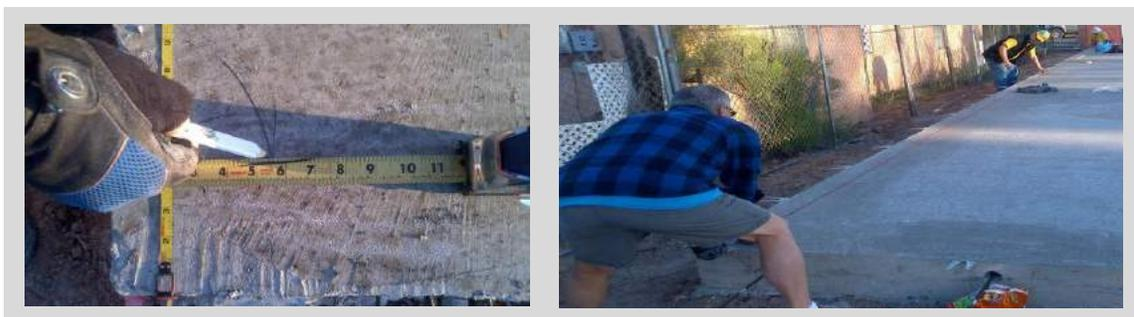
2. Lay out all exterior walls parallel to your control line by measuring from the control line to each end of each of the parallel lines. Determine the length of each line and snap out only that length.
