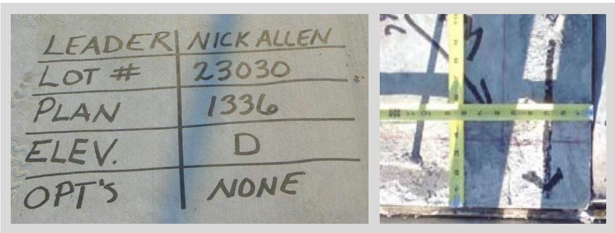
Typically, longer walls and walls with doors run long because you do not want to create a hinge point. Mark these walls on the slab with arrows as shown above right.
