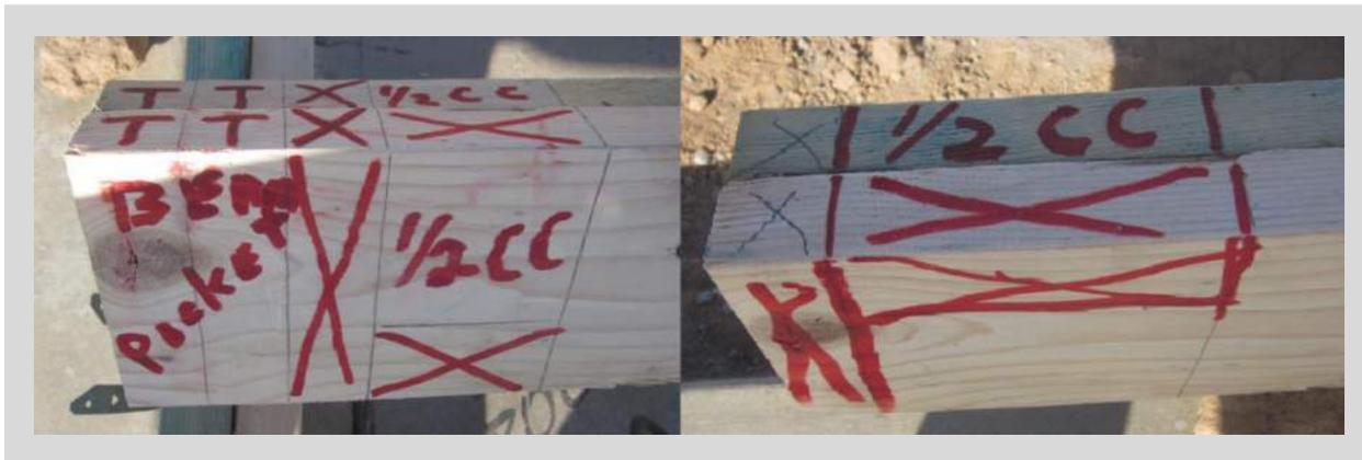
marks with a red marker and write “Beam Pocket” on top of the plates (see the above picture on the left).
