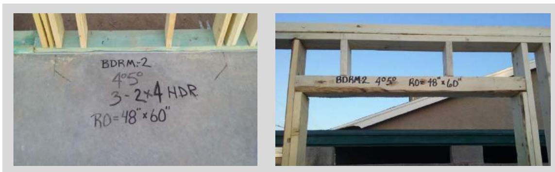
Plate breaks should be marked at this time. Locate the plate breaks on all exterior walls that are longer than 16'-0". They are to be placed at 16'-0" from the corner, and at every multiple of 16'-0" for the length of the wall. Mark medicine cabinet, tub backing and beam pocket locations on the slab.
